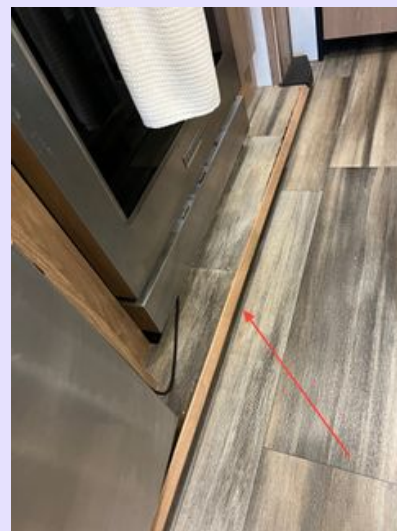
Trim under the Range and the Refrigerator.
