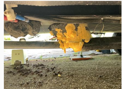
Additional foam added
