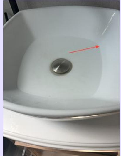
Main bathroom sink drains very slowly OBJ
