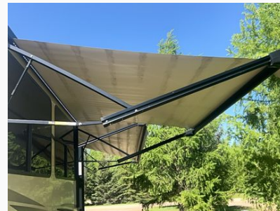
Discoloration on the inside of the awning.
